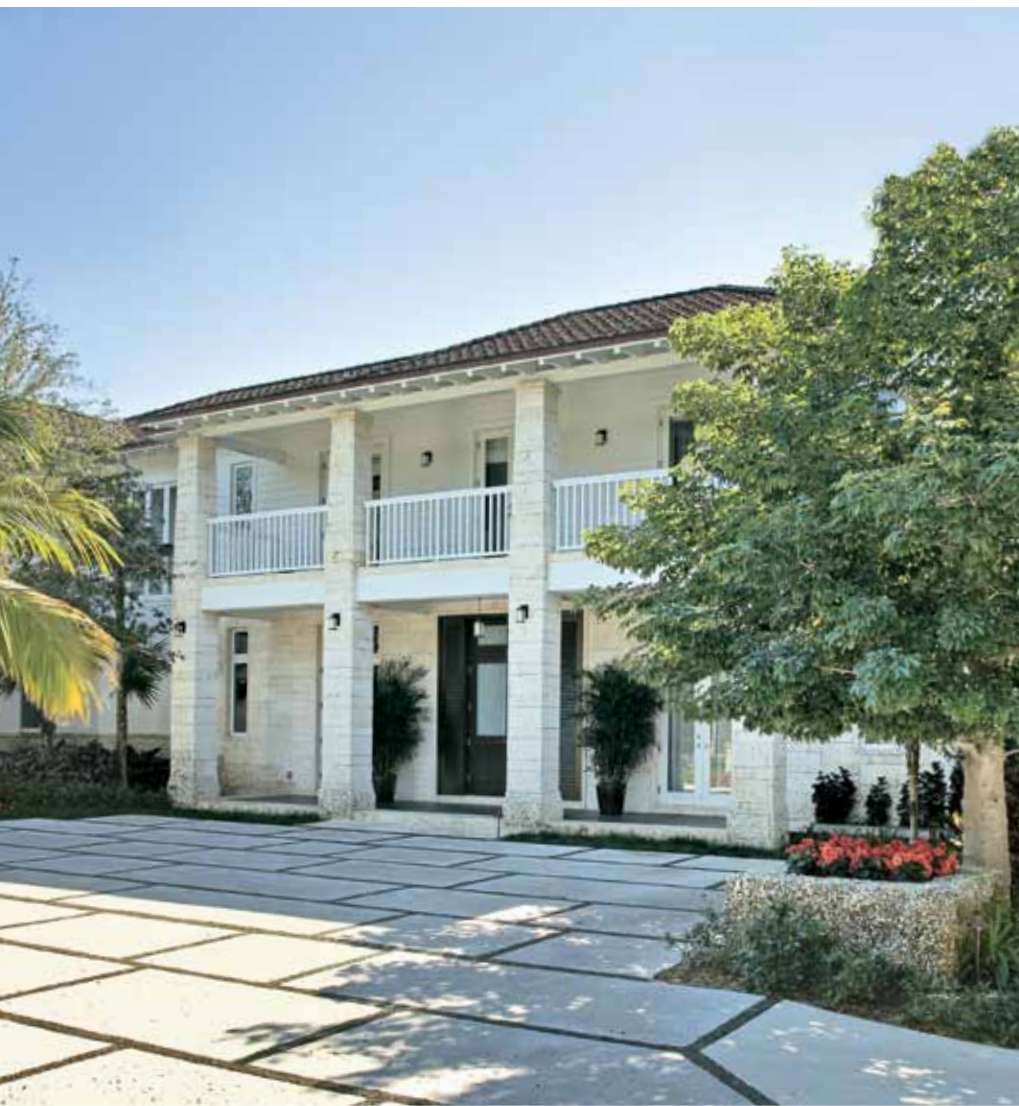
The house evokes a West Indies plantation home, with large windows, covered verandas, columns, and lush tropical landscaping. Natural oolite shell stone was quarried from the site and used as decorative cladding on the house. Madera split tiles on the roof mimic wood shingles.
